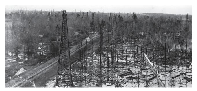
More than 75 derricks are shown drilling the field in Smackover, Arkansas, 1925. The large number of wells drilled too closely together caused damage to the natural resources above and below the surface. Arkansas Museum of Natural Resources (1985.016.001).
