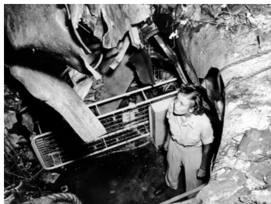
Photographed at Guam, Army Nurse First Lieutenant Mary Jensen of San Diego, California, looks up through the hole in the concrete and steel deck of the Navy hospital ship Comfort , May 3, 1945. Courtesy of the National Museum of the Pacific War.
