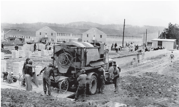
Early construction of the laboratory building behind Manhattan Engineering District Administration Building in Oak Ridge, Tennessee, 1943. US Department of Energy/Ed Wescott 2/16/1943.
